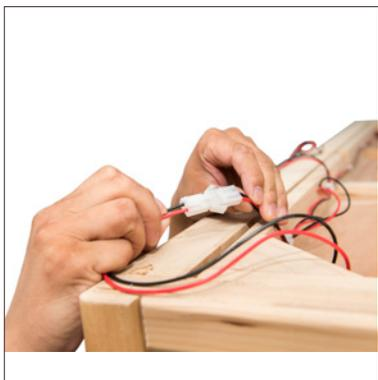
Connect all the lights to the cables already on the roof. You must connect the 2 top lights, the LED strips for chromotherapy as well as the light under the bench.
