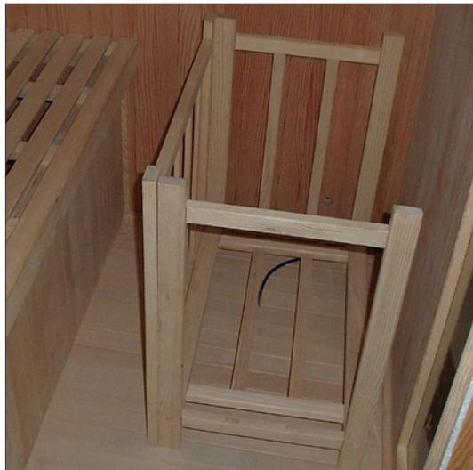
The stove's protective cage must be assembled then installed inside the cabin.
